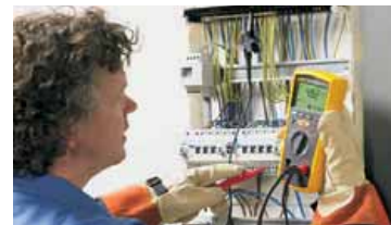
Insulation test at a distribution panel
